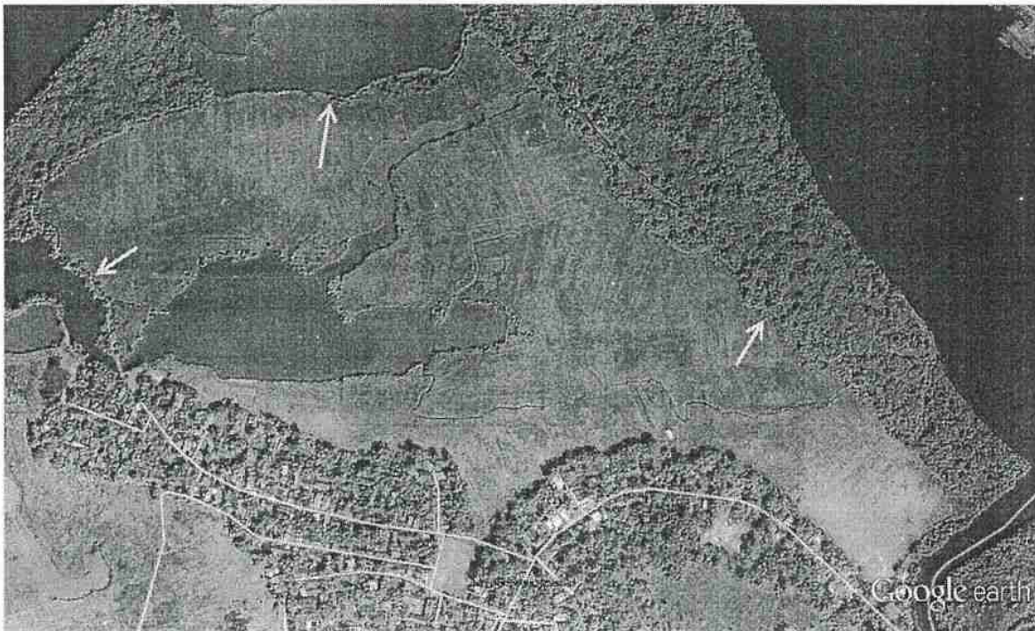
GE image 12/2013: The Cavso Cantor bundh as it appeared before the embankment was reclaimed; the entire wetland complex presents a natural landscape; the embankment marked by a continuous mangrove fringe can be faintly seen (shown by arrows in yellow).
