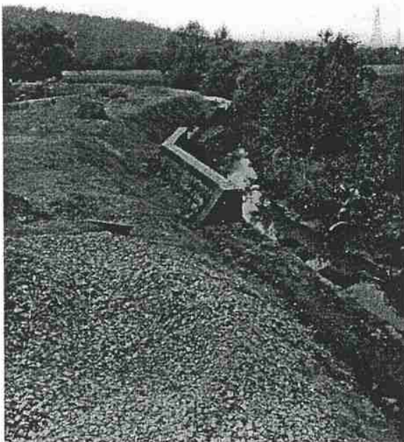
Left: About 100 metres from Cupa sluice gate; work on the rubble – concrete wall along the widened embankment; here, the embankment would be 6-7 metres wide, and about one metre above high tide level; mangrove fringe is still seen. Right: The trunk of a mangrove that is cut; smaller mangroves seen in the background.
